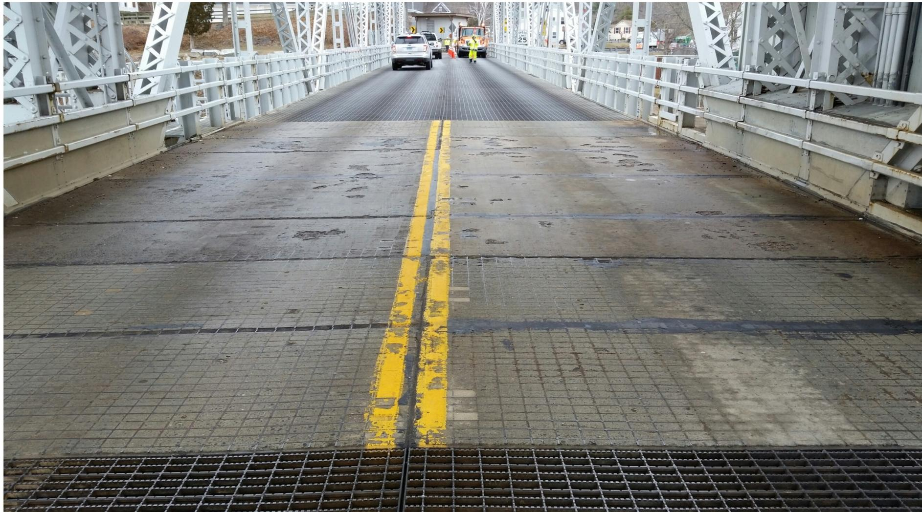
Concrete Filled Grid Deck Over Center Equipment Room
